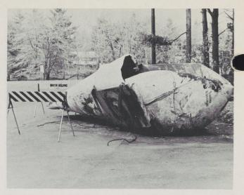
Front portion of T-24's cargo tank after being moved from its position in the woods.
